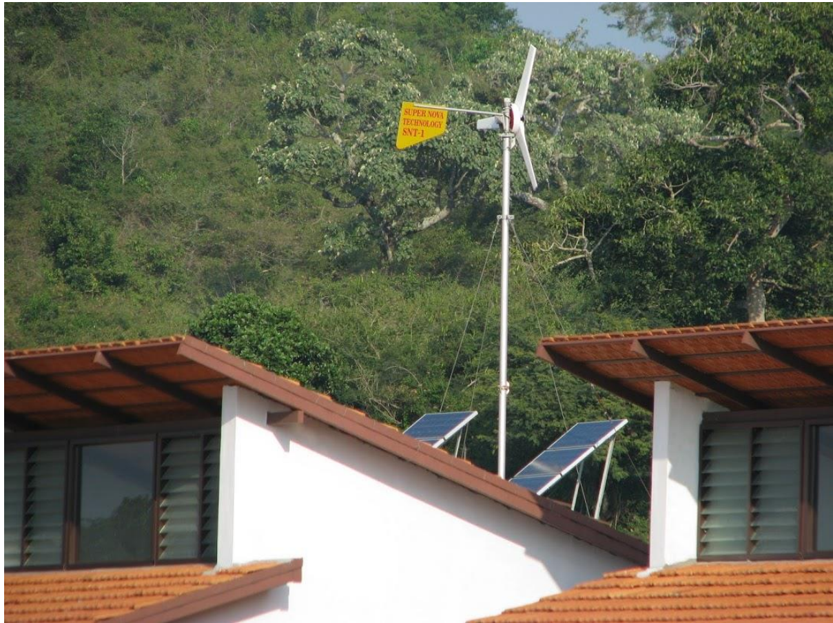
Combined wind and solar generation at Dhole's Den.
