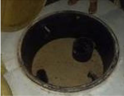
Grease traps are good practice to prevent oil and grease from entering water treatment systems and creating problems. The process is cost effective and requires very little investment. Pictured here grease trap behind the kitchen at Limban Resort.
