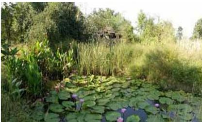
A DEWATS reed bed system is used to filter grey water from the kitchen at Forsyth Lodge. Grey water from guest cottages passes through filtration pits to a lily pond. A septic tank is used to treat black (sewage) water. Read case study.
