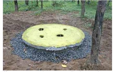
Five new recharge wells have been installed at Singinawa Jungle Lodge with a depth of 10 ft, diameter 5 ft and capacity of 250 cubic metres per year to harvest rain and recharge groundwater.
