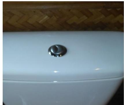
Dual-flush toilets, in use by numerous PUG rated lodges, are also positive for saving water. The best models use only 3-6 litres per flush compared to 10-13 litres in single flush models while still achieving equal or superior performance.
