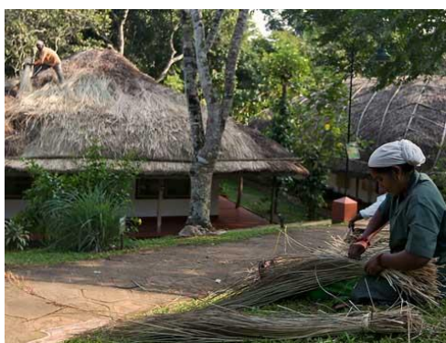
Buildings have wide eaves for natural cooling and are thatched with elephant grass annually.
