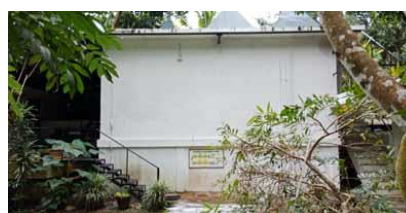
A sewage treatment plant and an effluent treatment plant is in place enabling 45 kl of water to be recycled daily.
