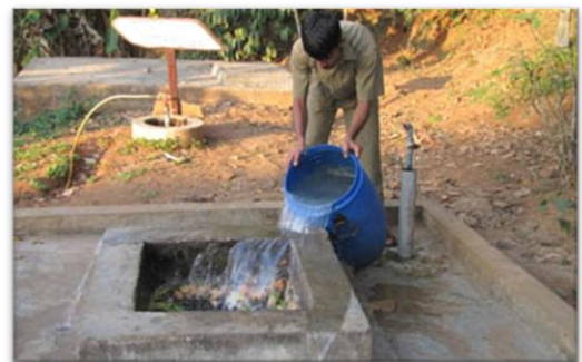
Biogas unit using food waste to power cooking.
