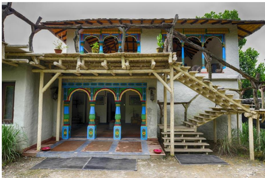
Buildings reflect local Kumaoni traditions using local materials and labour.
