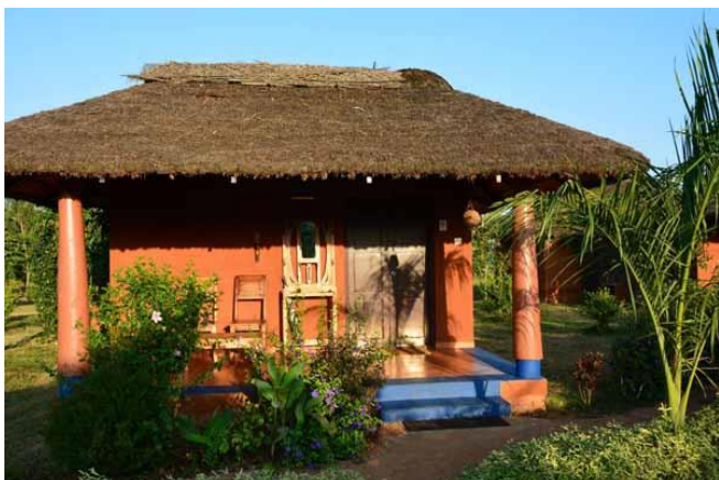
Cottage built with traditional rammed earth technique and elephant grass.
